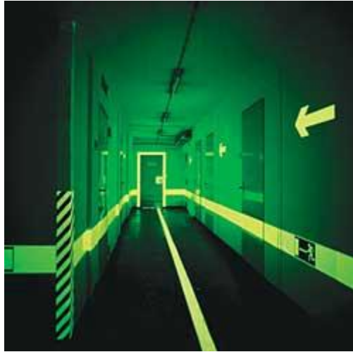
Figure 11.1 – The use of fluorescent paint along escape routes can be an effective aid
